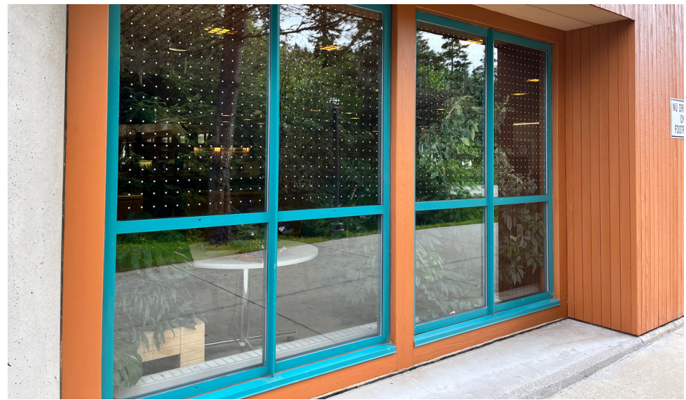
Anti-collision retrofit on windows at the Egan Library. Photo: Courtesy UAS
